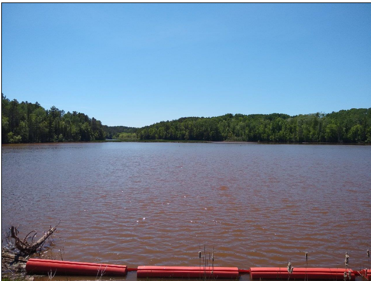
Figure 4.9.1-1: View Upstream from the White River Dam
